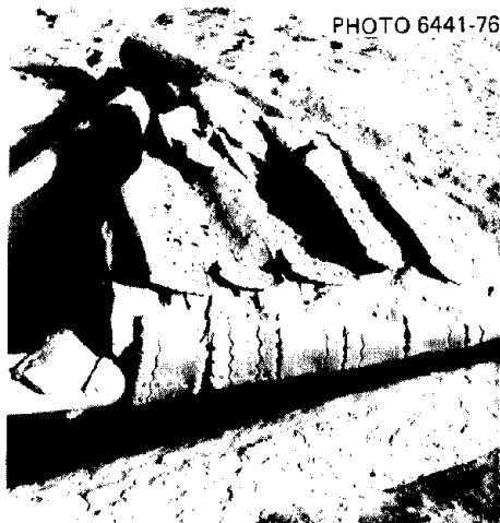
Fig. 6.6. Posttest condition of expedient triangular blast door. Some flap valves had been jammed shut, and much earth and sand had been deposited.
